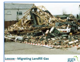
Loscoe - Migrating Landfill Gas
